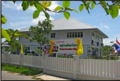
Main Building & Sign Board
